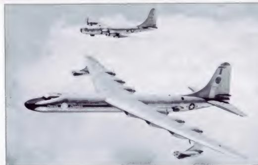
The NB-36H carried a nuclear reactor to test its effect on the aircraft. The next step would have been a nuclear-powered bomber.
